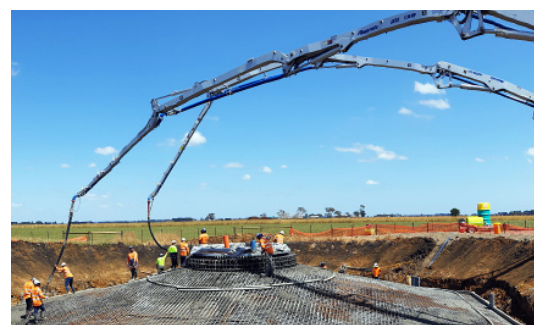
Mortlake South Wind Farm ▲ (under construction)
