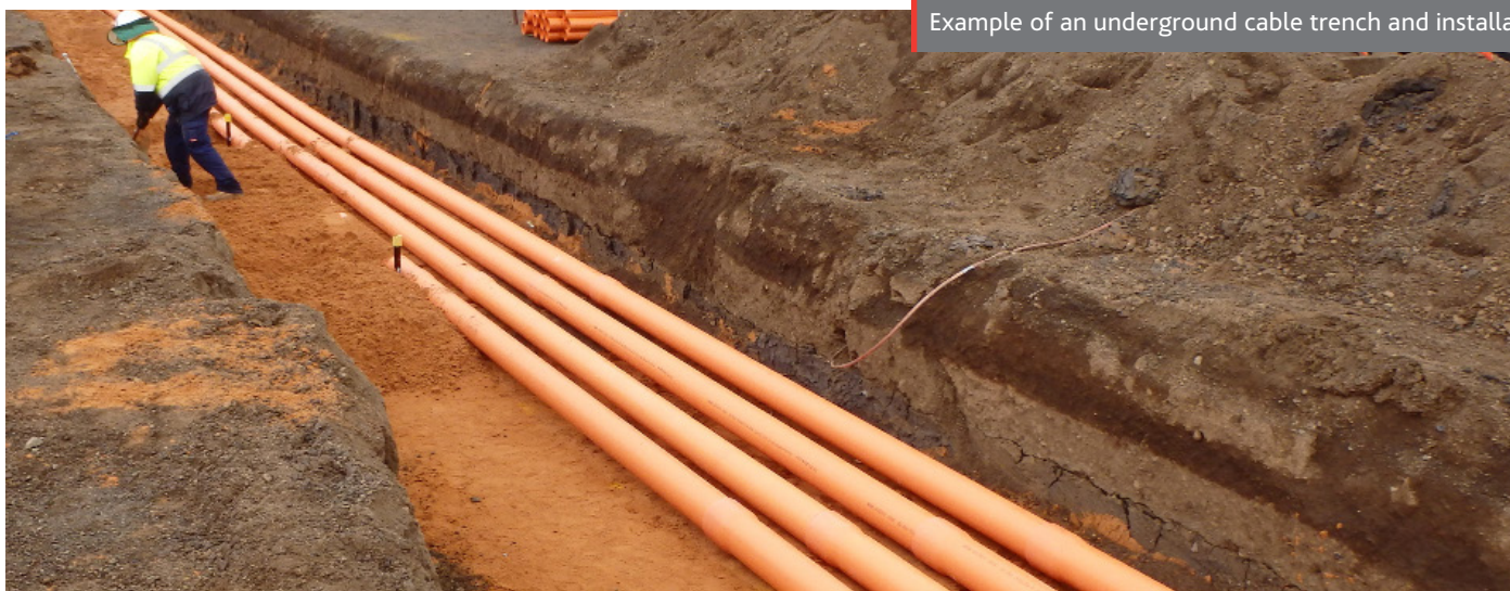
Example of an underground cable trench and installation
