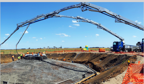
▲ Mortlake South Wind Farm, VIC (under construction)
