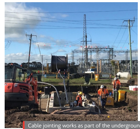
Cable jointing works as part of the underground connection line installation
