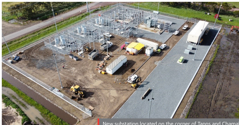
New substation located on the corner of Tapps and Chamallak Lanes
