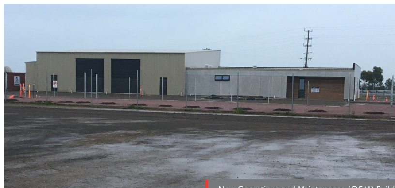
New Operations and Maintenance (O&M) Building
