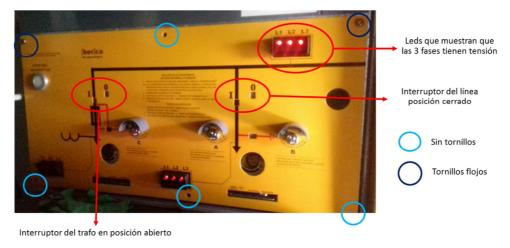
Close-up showing the condition in which the switchgear panel was found.
