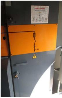
Close-up of the contactor switchgear panel door. The interlock keys (B and C) are correctly inserted into their locks.
