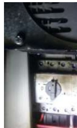
Close-up of the TOP cabinet and motor protection breaker FG380, where the arc was produced.
