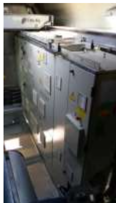
Close-up of the TOP cabinet and motor protection breaker FG380, where the arc was produced.
