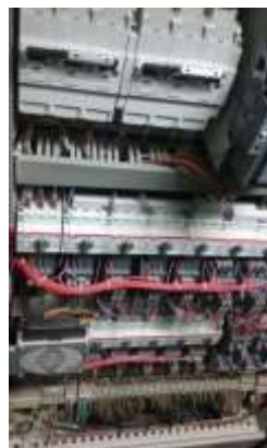
Close-up of the TOP cabinet and motor protection breaker FG380, where the arc was produced.
