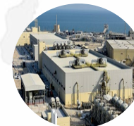
Al Khobar I desalination plant Saudi Arabia
